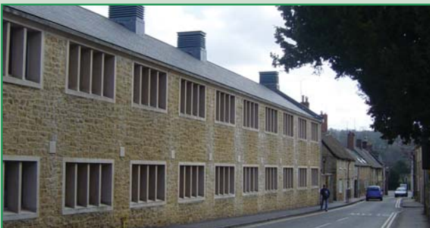
Contemporary chimney vents in new build, Sherborne
