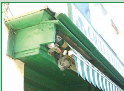
Traditional blind mechanism
