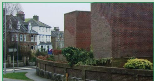
Lack of any detailing or interest is unacceptable
