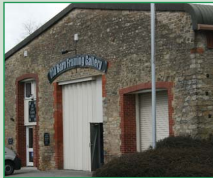
Industrial converted stone building with modern metal roof, Sherborne
