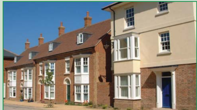
Example of detailing at Poundbury
