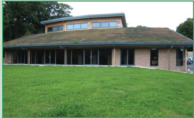
Green roof at Kingston Maurward
