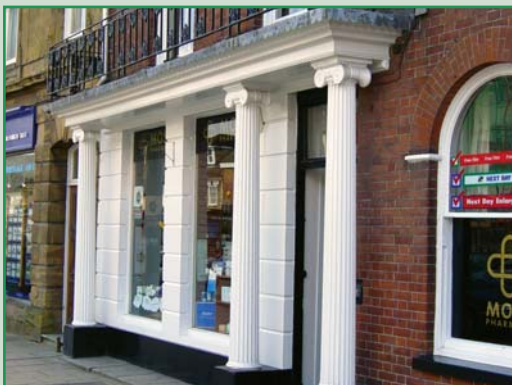
c) Regency shopfront, Bridport
