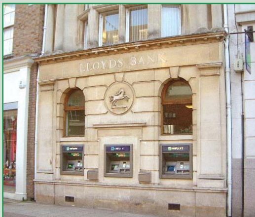
Cashpoint integrated into window design
