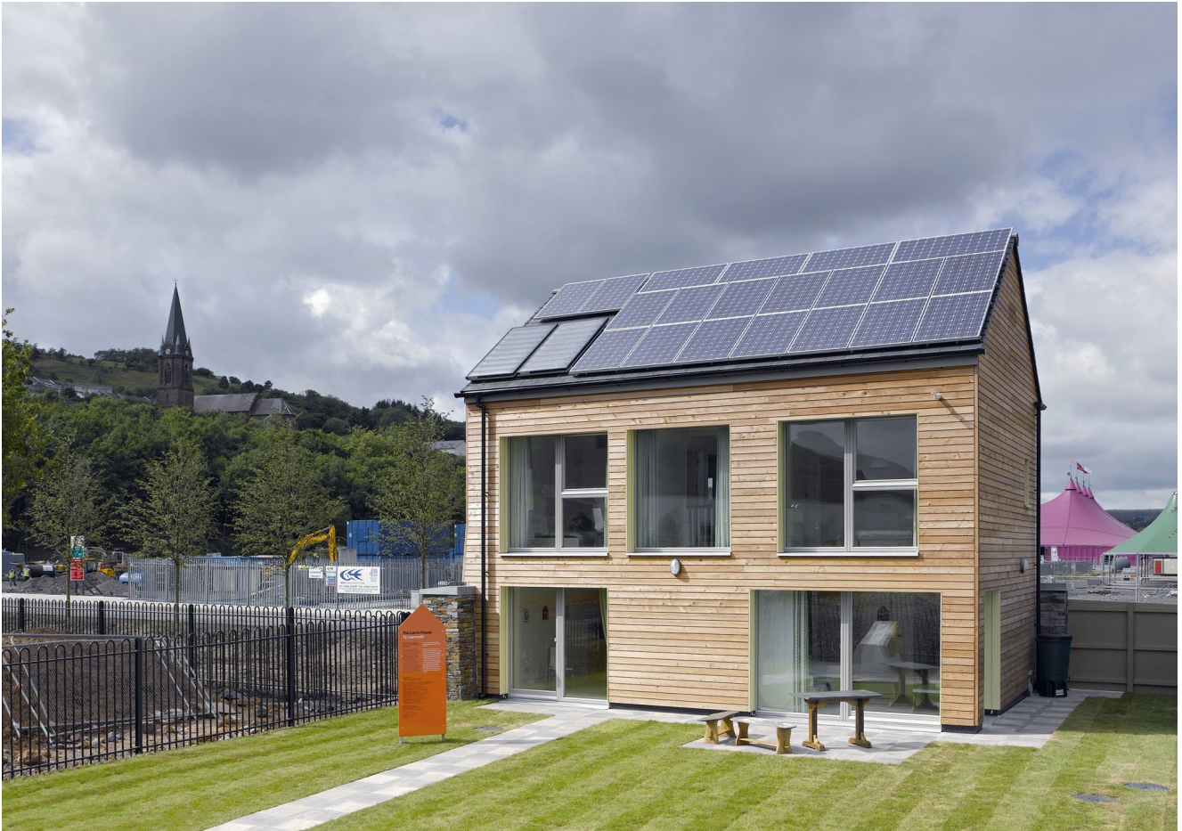
Bere Architects award-winning Larch House
