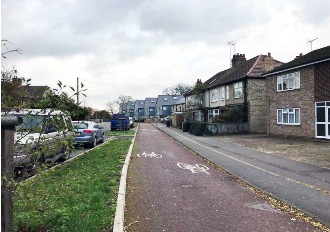
Example of fully Kerbed Segregated Cycle track and pedestrian route
