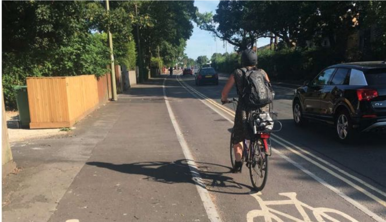
Example of 'half kerb height' construction
